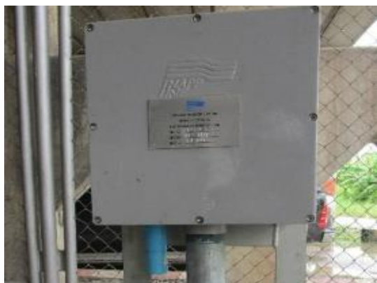
Cathodic Protection System
